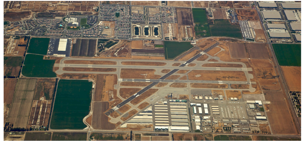
Issues arriving from land acquisition and construction are common impediments to airport expansion.
